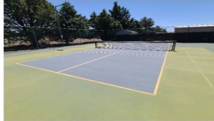
PICKLEBALL COURTS WILL BE RESURFACED
