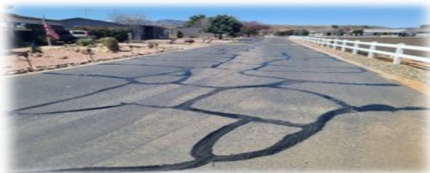
CRACK FILL FOR ALL ROADS NOT REPLACED
