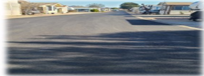
ROAD REMOVAL AND REPLACEMENT
