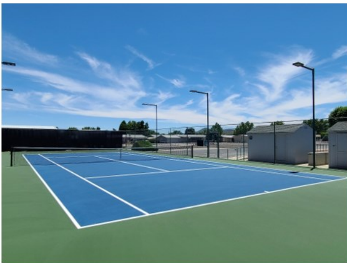
TENNIS COURT RESURFACED
