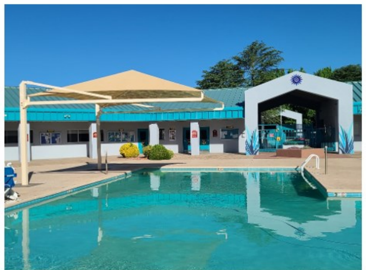
NEW POOL SHADE COMPLETED
